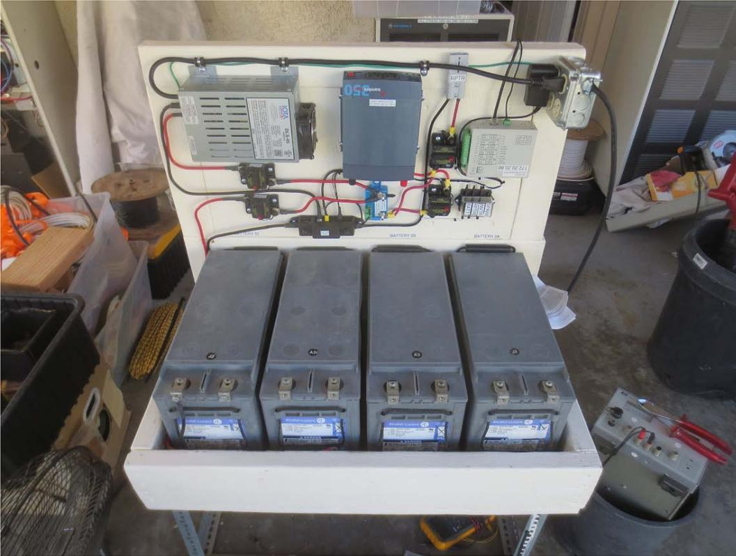
The long awaited battery backup system was installed today. The system provides 560 amp hours of battery from four each 140 amp hour batteries (105 lbs each) a 45 amp power supply/charger, 110volt pure sine wave inverter and a remote telemetry monitoring system.
