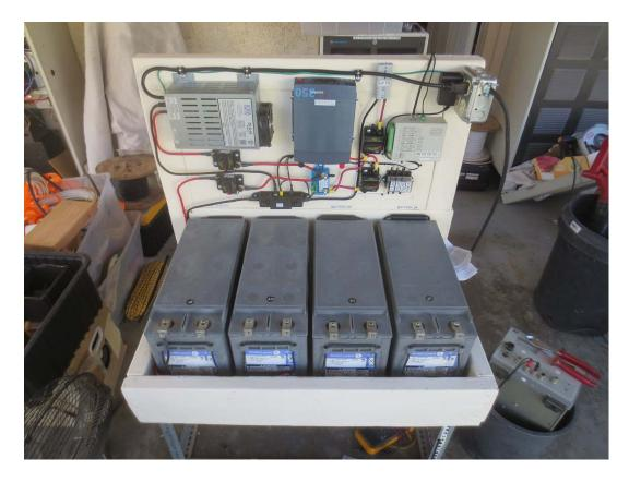
The long awaited battery backup system was installed today. The system provides 560 amp hours of battery from four each 140 amp hour batteries (105 lbs each) a 45 amp power supply/charger, 110volt pure sine wave inverter and a remote telemetry monitoring system.
