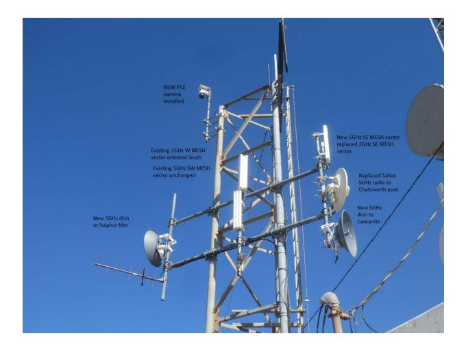
Getting back to the October 29th trip, this day saw the addition of a Pan Tilt Zoom camera, replacement of the 2GHz SE Mesh sector radio/antenna with a 5GHz SE Mesh sector radio/antenna and realignment of the 2GHz Mesh sector radio/antenna from SW to S.
