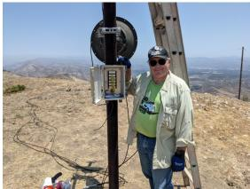
The network connectors were installed at the remote network location and plugged into the network lightning protection panel. Once completed the remote team members departed the hilltop. Excellent work by all!
